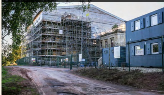
House restoration Gradually returning to its former glory
