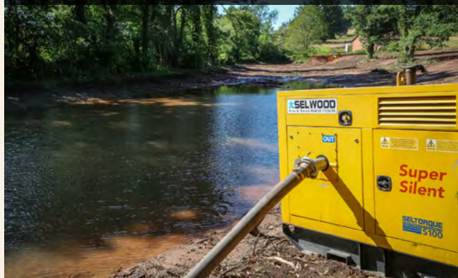
Lakes The parkland lakes are being dredged and re-established
